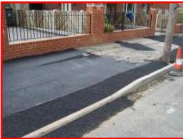
**Refurbishment** – Typically this includes all elements (kerb, footway and carriageway) being treated to varying degrees. The kerbs may require isolated repairs or the full length will either be relayed or replaced with new kerbs. The footway and carriageway will either be covered with new material or the existing surface will be removed and replaced (as described above).
