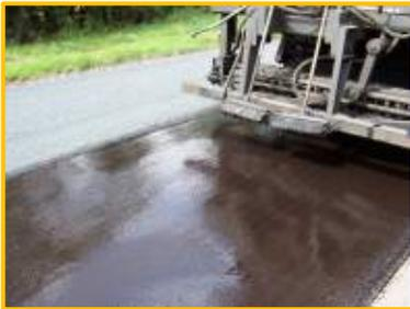
**Surface Dressing** – Any defects in the carriageway are repaired ahead of the treatment. The road is then sprayed with a hot bitumen binder. This softens the road and seals the existing road. A layer of new stone chippings will then be spread over it and rolled. Because the surface is soft the chippings will bed into the binder and the existing surface. This will continue over the next few weeks under the normal traffic action.
