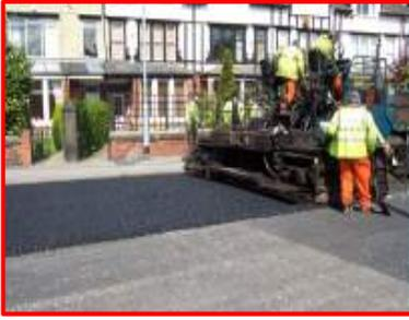
**Reconstruction** - This is the most expensive type of treatment and usually involves replacing the surface course, binder course and base with new materials.
