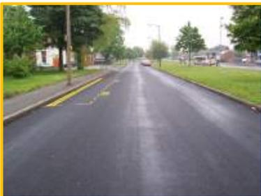
**Micro Asphalt** – Any defects in the carriageway are repaired ahead of the treatment. It is usually laid in two layers, the first layer to fill any defects and regulate out any dips in the surface. The second layer provides the new surface. Micro Asphalt is laid as an emulsion, a mixture of bitumen mixed with crushed stone. It is laid cold and stays liquid for about 20 minutes before it sets (hardens) at which point the road can be opened to traffic.
