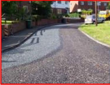
**Recycling** - The road is broken up and new bitumen is added, these are then mixed together and the material can be reshaped and rolled to create a solid structural layer. The surface is then sealed with a surface dressing. It is also known as 'Retread' - Shallow In-Situ Recycling because it only goes down 75mm (3") and 'in-situ' because the material is recycled on site.
