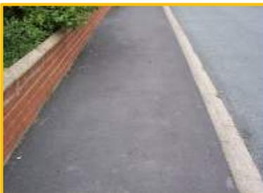
**Footway Surface Treatment (Slurry seal)** – This involves the laying a thin layer of bitumen mixed with crushed stone over the top of the existing footway to seal the surface and extend its life.
