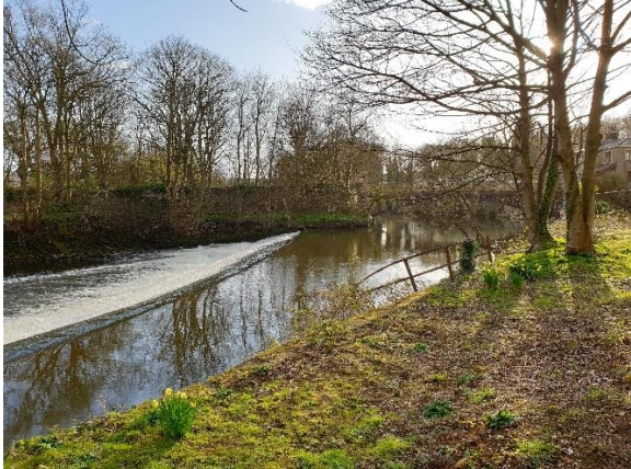
Figure 3: SW to Newlay Weir and Newlay Bridge.
