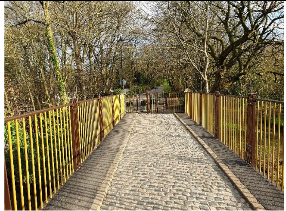
Figure 2: SE from Newlay Bridge to Pollard Lane.
