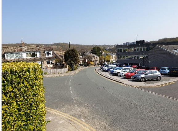
Figure 27: Due S to Woodside Methodist Church from Outwood Lane. Woodside Quarry in distance.
