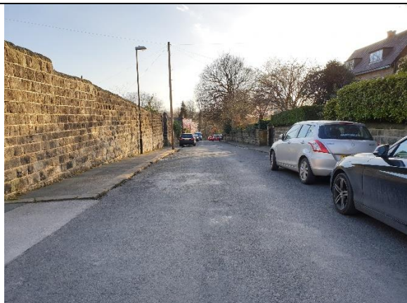
Figure 14: SW on Clarence Road.
